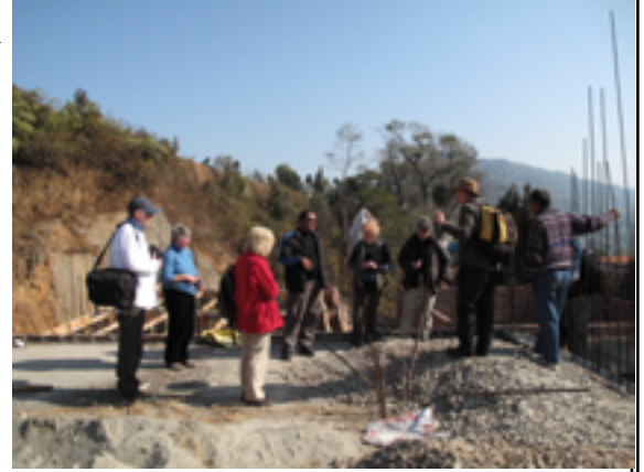
Kalimpong workshop construction site
