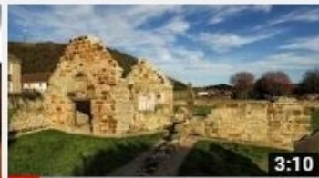
Kirkton Church Restoration Project
